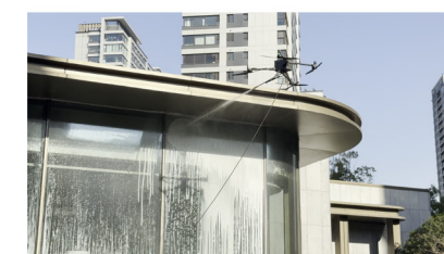
Drone-based Exterior Wall Cleaning
